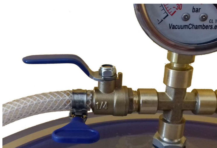
Photo 8: Pneumatic hose mounted on the barb of the ball valve, secured with worm drive hose clamp.
