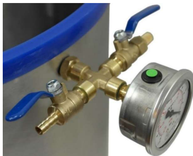
Photo 6: Air manifold correctly installed.
